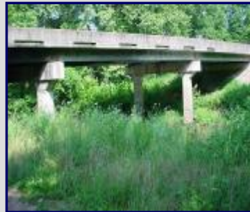
View of the Dallas County Bridge, MO
