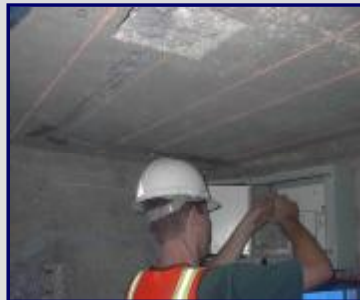
Fiber Optic Installment for Strain Measurements
