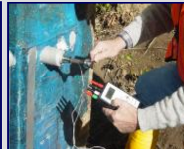
Bond Str. Measurements by Pull-out Tests
