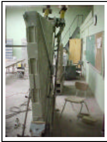
Figure 8. Slope for the Out-of-Plane phase in one-side reinforced walls
