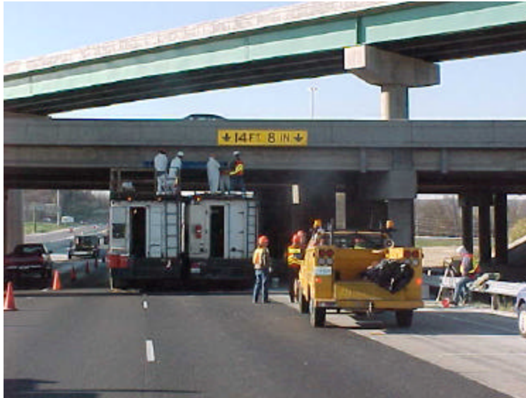
Figure 5. Installation Crew at Work
