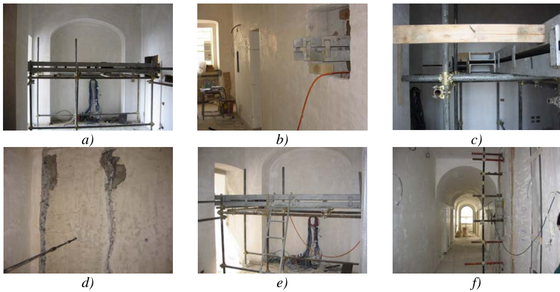
Figure 6 - Pictures of the Test Setup
