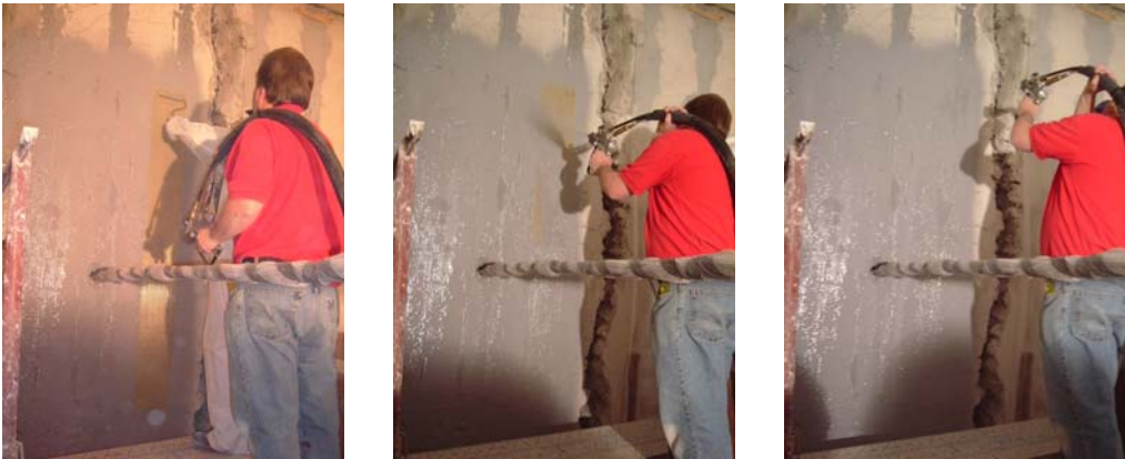
Figure 2 - Pictures of the Strengthening Phase
